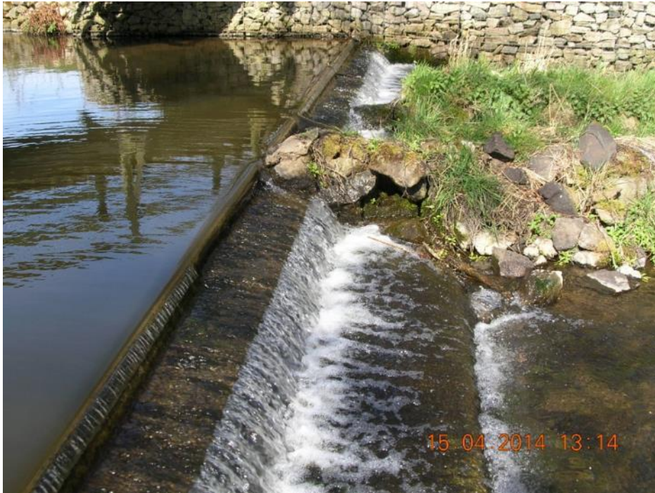
NORTH EAST OUTFALL WEIR. APRIL 2014.
