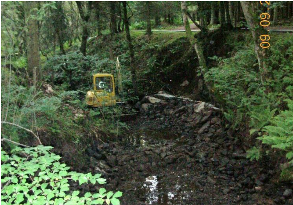
BANK REINFORCEMENT NEARLY COMPLETE.
