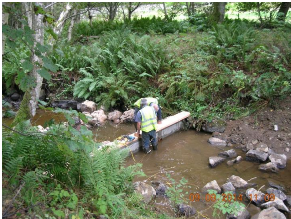
SECOND PRE WEIR NEARLY COMPLETE.
