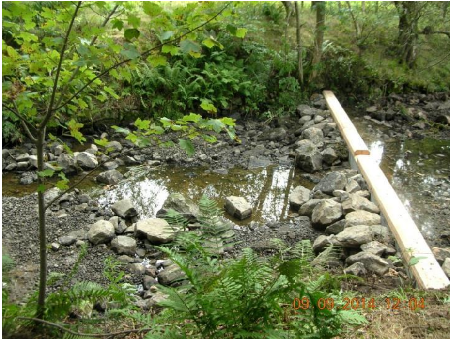
UPPERMOST PRE WEIR COMPLETE.
