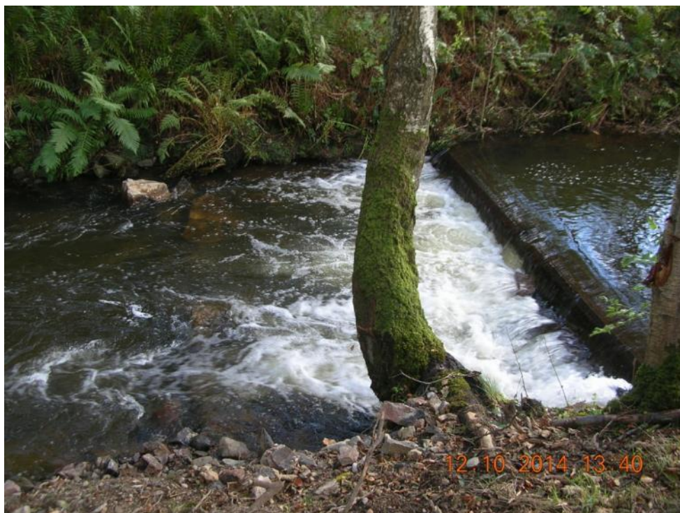
NEW SECOND PRE WEIR AND BOULDER PLACEMENT.
