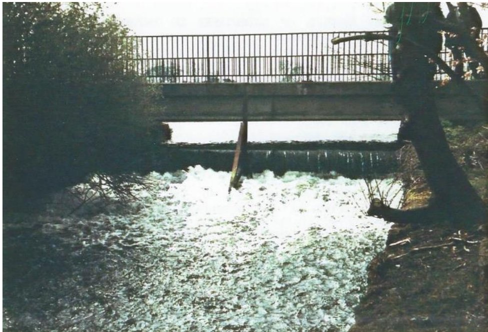
NORTH CENTRAL OUTFALL WEIR. 1986
