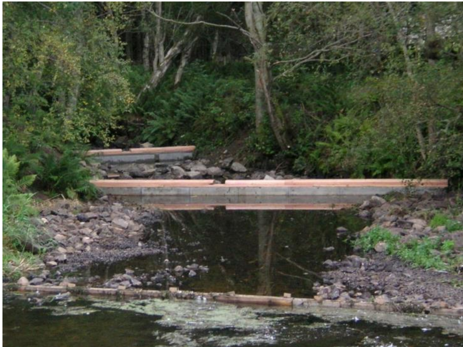
DOWNSTREAM VIEW. WEIRS COMPLETE.
