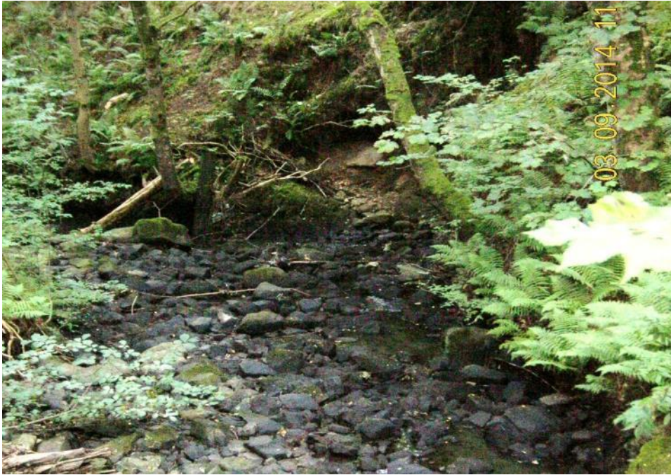
VIEW DOWNSTREAM OF LOWER FALL, SHOWING SERIOUS EROSION OF RIGHT BANK.
