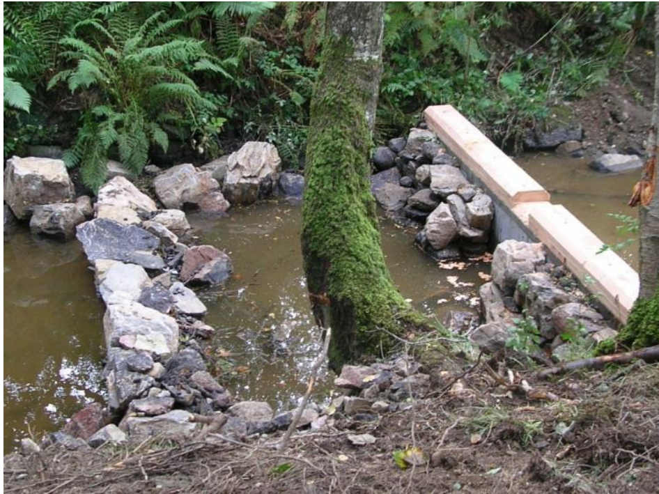
SECOND PRE WEIR AND BOULDER PLACEMENT BELOW.
