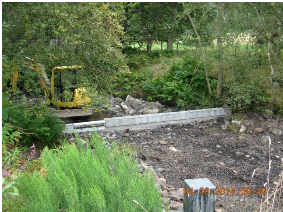
UPPERMOST PRE WEIR UNDER CONSTRUCTION.
