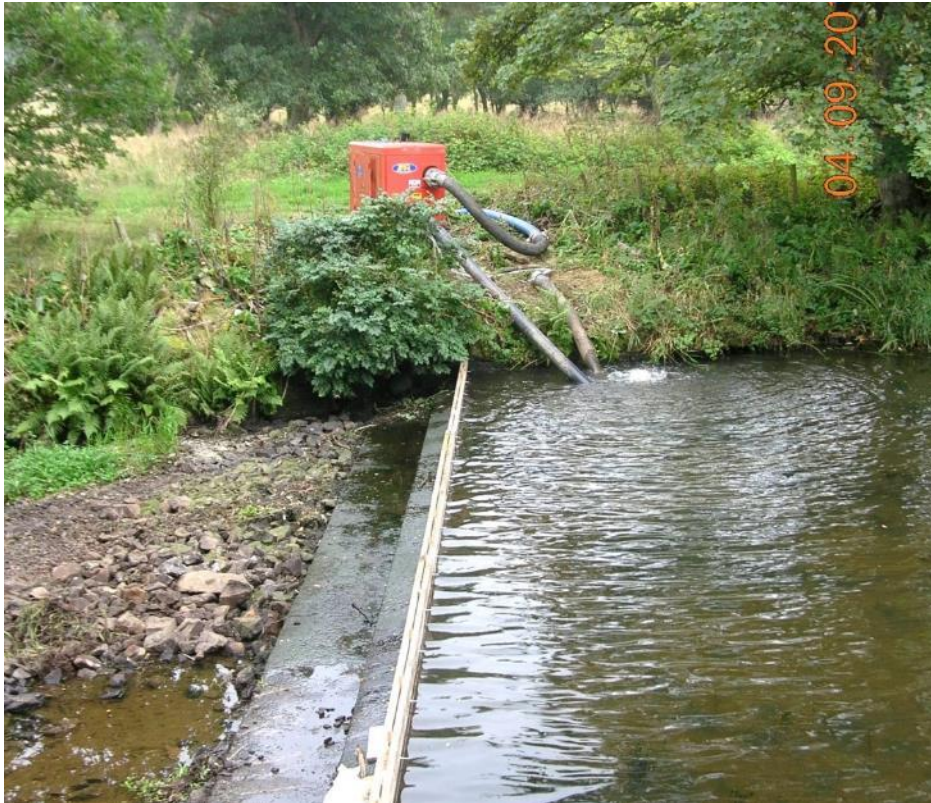
WEIR BLOCKED OFF AND PUMP OPERATING TO BYPASS THE WORK AREA.
